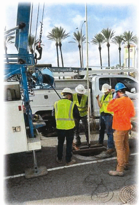
Rehabilitation Conducted on a Monitoring Well
